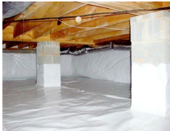
Closed (sealed) Crawlspace
