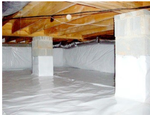
Closed (sealed) Crawlspace
